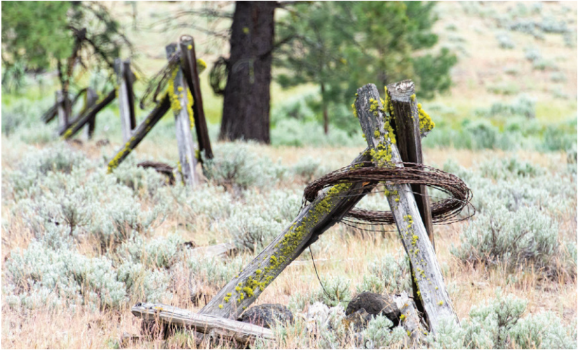
Removal of unneeded fencing
